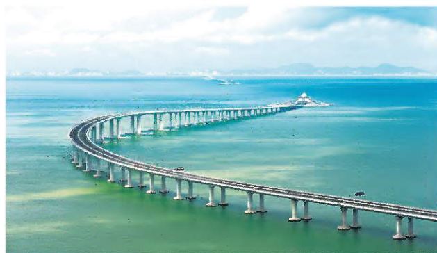
The 55-kilometer Hong Kong-Zhuhai-Macao Bridge is the longest bridge-tunnel sea crossing in the world.
